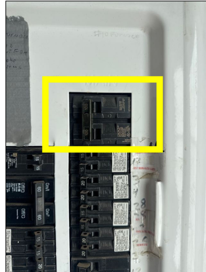
Main electrical shut off inside the sub panel.
