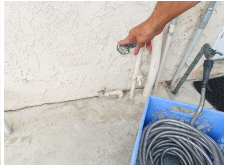
some hose bibs have no water when testing
