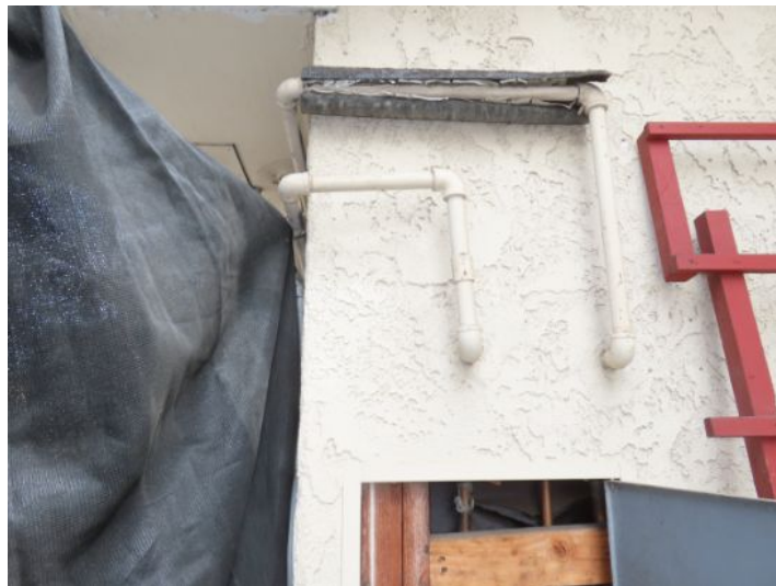
exterior plumbing present at the west side to the bathroom
