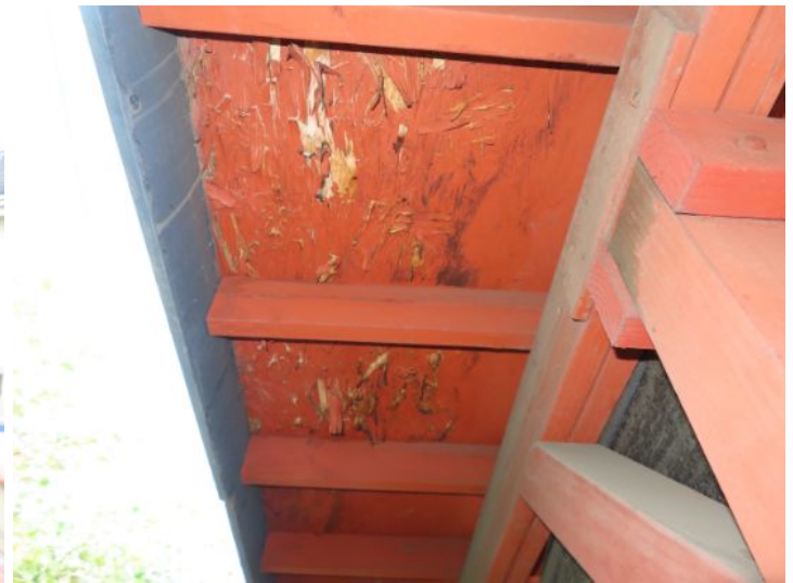
deteriorated wood
