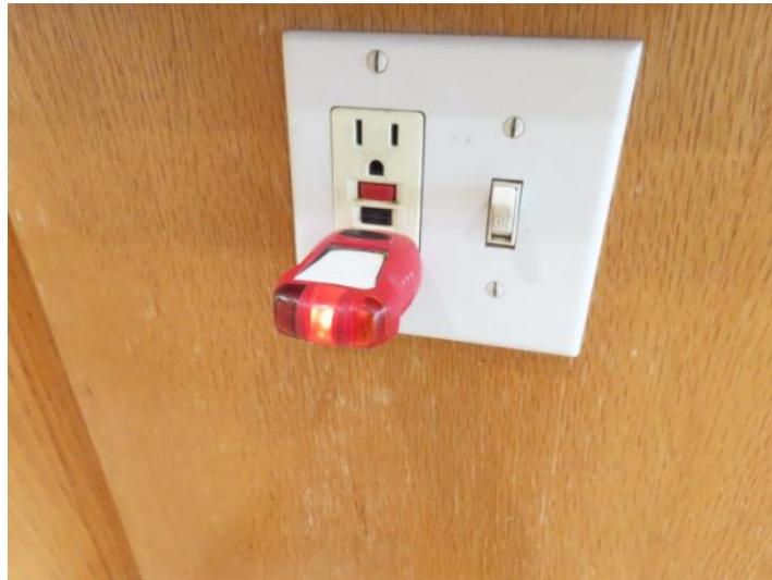
GFCI outlet is not grounded, test did not operate at the island
