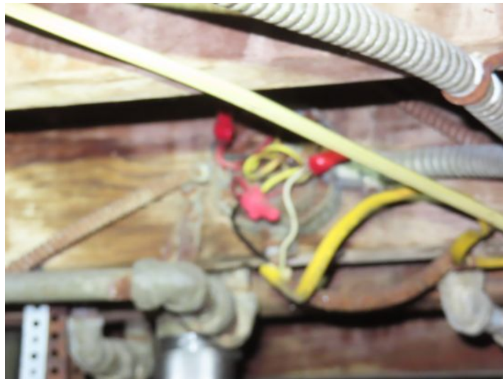
exposed connections
