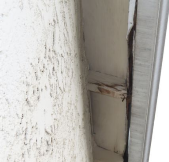
deteriorated wood
