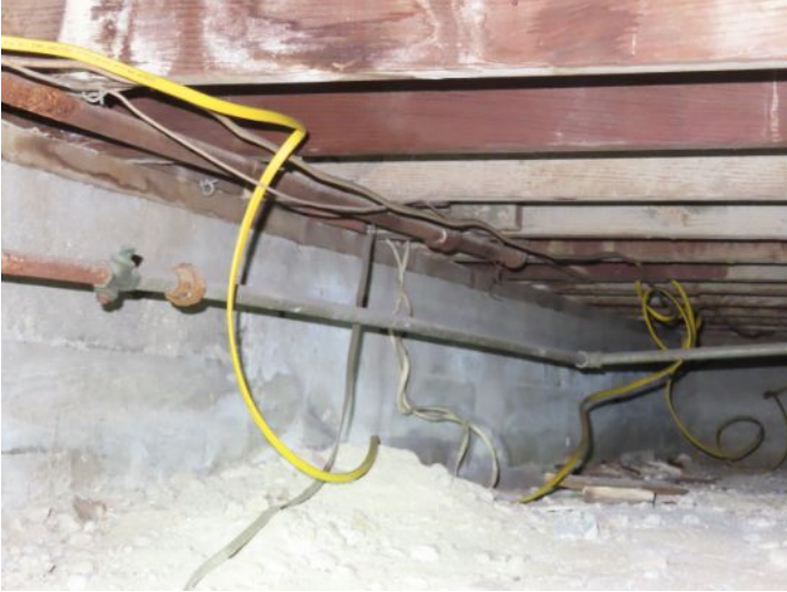
unsecured wiring
