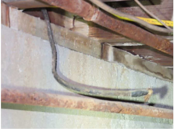
exposed wires
