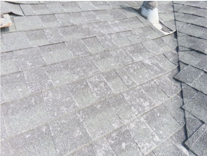
deteriorated roofing material
