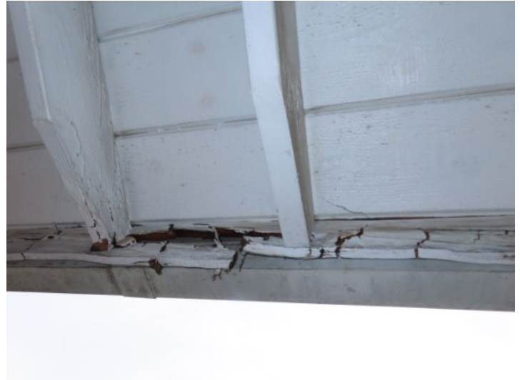
deteriorated wood
