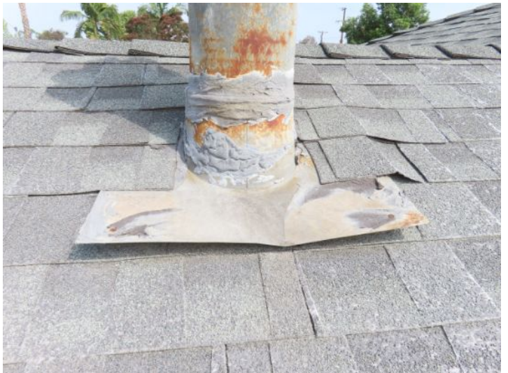
lifting metal flashings
