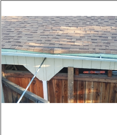
Metal roof installed beneath roof shingles
