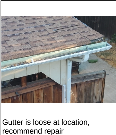
Gutter is loose at location, recommend repair
