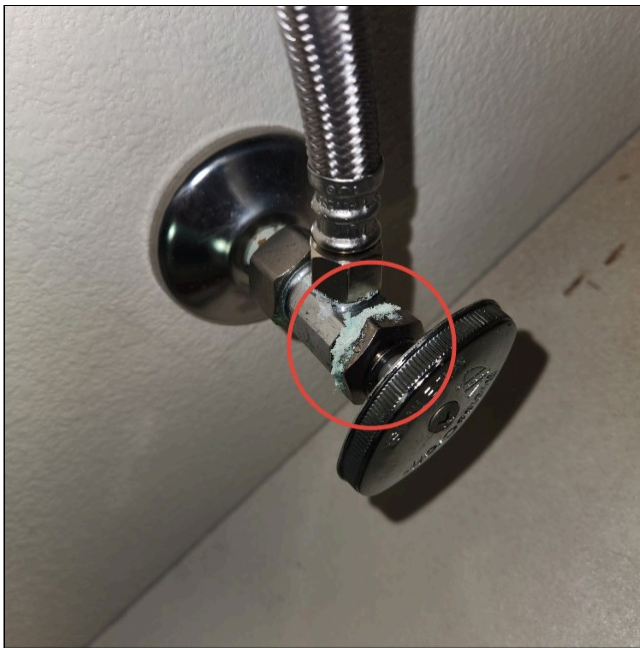
Corrosion/Mineral Deposits
