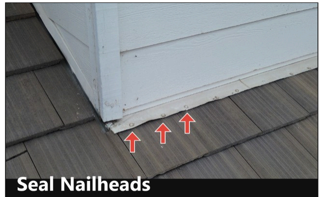
1.1 EXPOSED FLASHING
