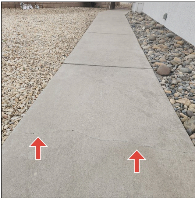
Seal Gaps/Cracks
