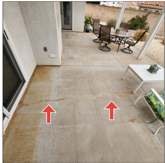
Seal Cracks
