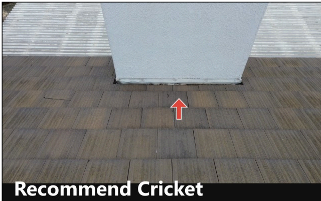
1.1 EXPOSED FLASHING
