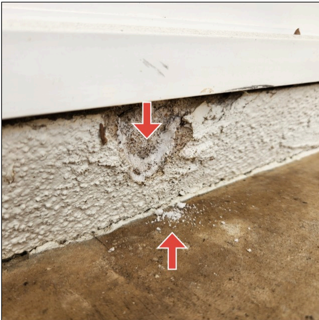
Efflorescence
