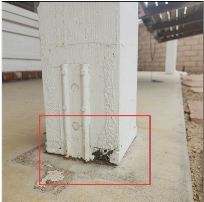
Wood Damage/Rot
