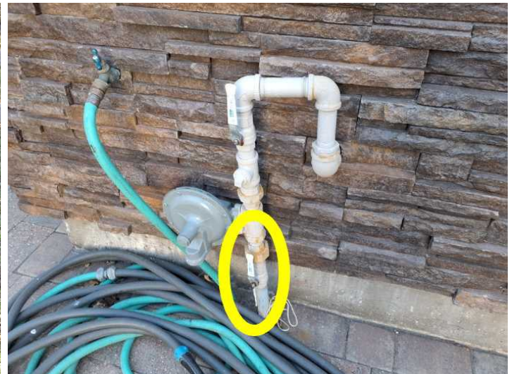
The local gas shut-off is located on the right side of the home, unit or building.
