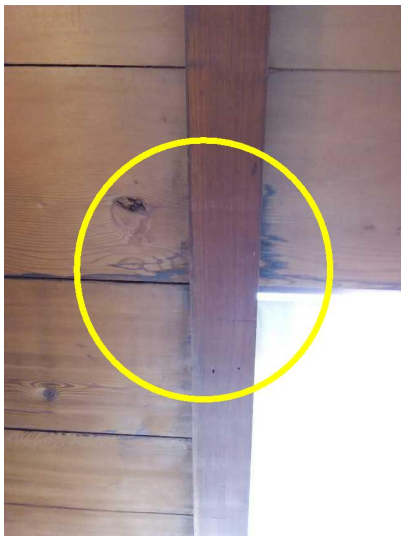
There is a moisture stain on the ceiling that should be explained or explored further.
