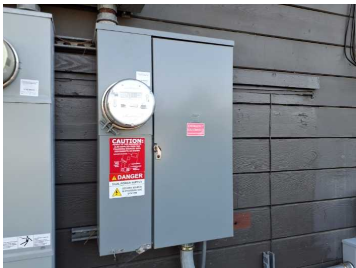
The residence is served by a 200 amp main electrical panel, located at the exterior of the office unit.
