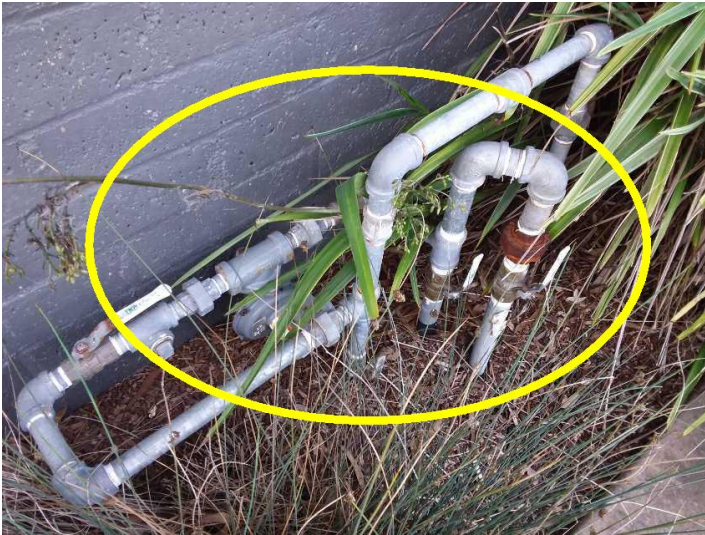
The gas main shut-off appears to be located on front of the home, unit or building.
