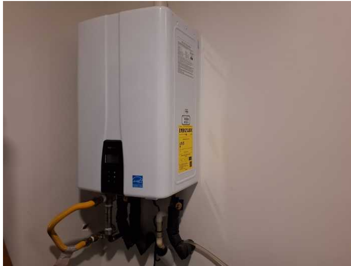
The residence is served by a tankless water heater located in the utility room.
