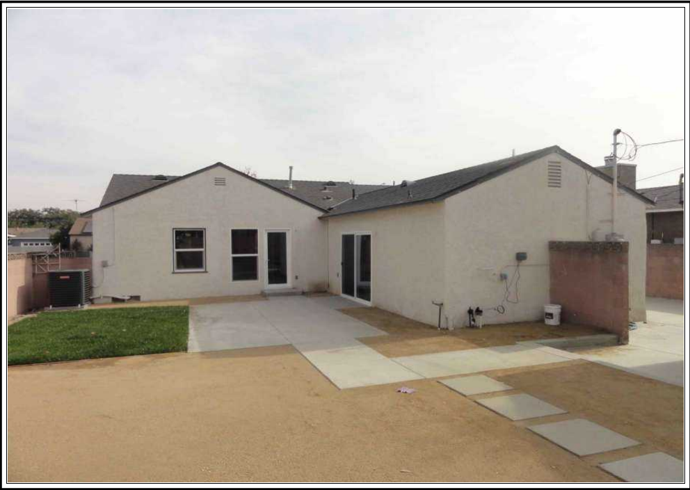
REAR OF SUBJECT PROPERTY
