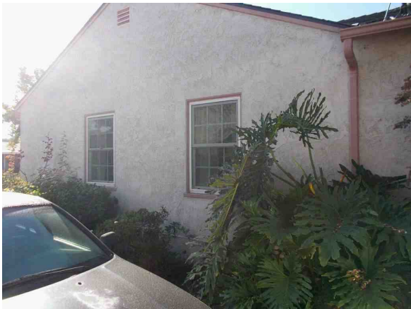
North Side From Rear
