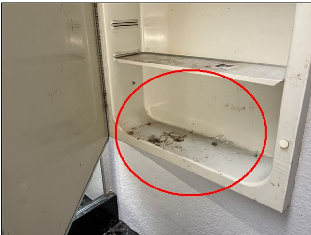
4.4 Item 3(Picture) primary bedroom bath: medicine cabinet oxidation visible
