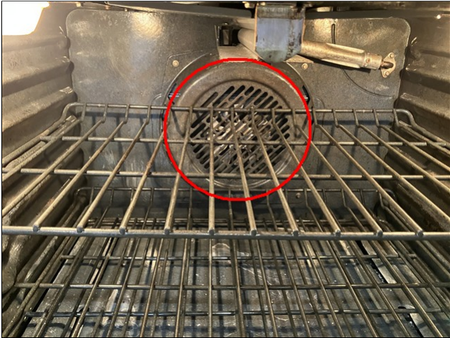
10.1 Item 1(Picture) convection fan did not turn on when tested
