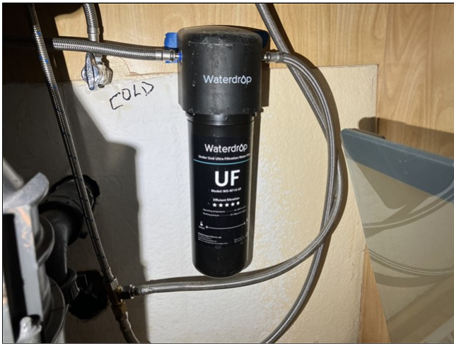
6.8 Item 1(Picture) kitchen: water filter was not inspected or tested as part of the scope of this inspection
