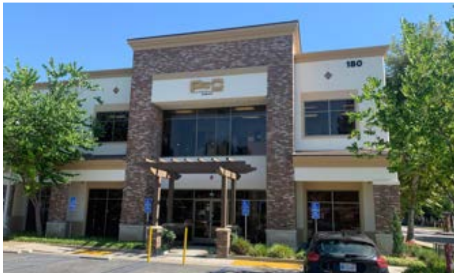
Massing accentuates main building entrance
