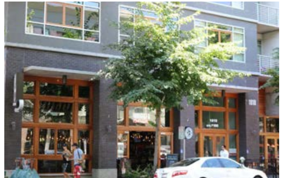
Mixed-use building showcasing harmonious high-quality materials
