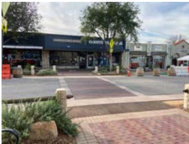
Mid-block crossing with decorative paving
