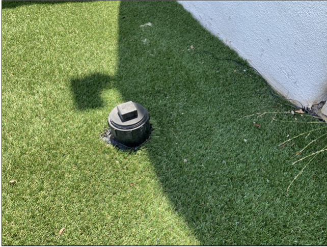
6.3 Item 3(Picture) 1817: sewer camera inspection recommended
