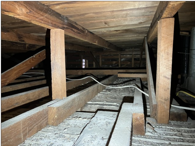
9.0 Item 1(Picture) 1819: insulation upgrades recommended
