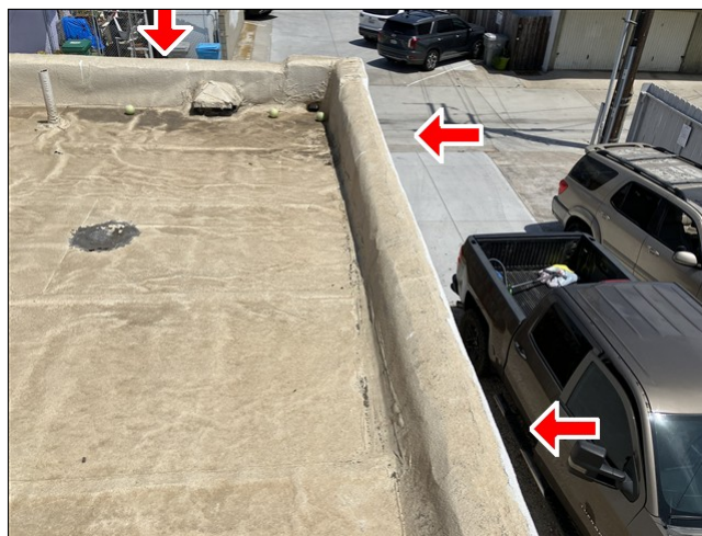
1.2 Item 2(Picture) 1819: parapet wall flashing caps recommended
