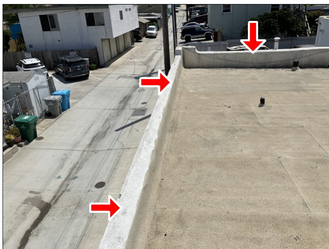
1.2 Item 1(Picture) 1819: parapet wall flashing caps recommended
