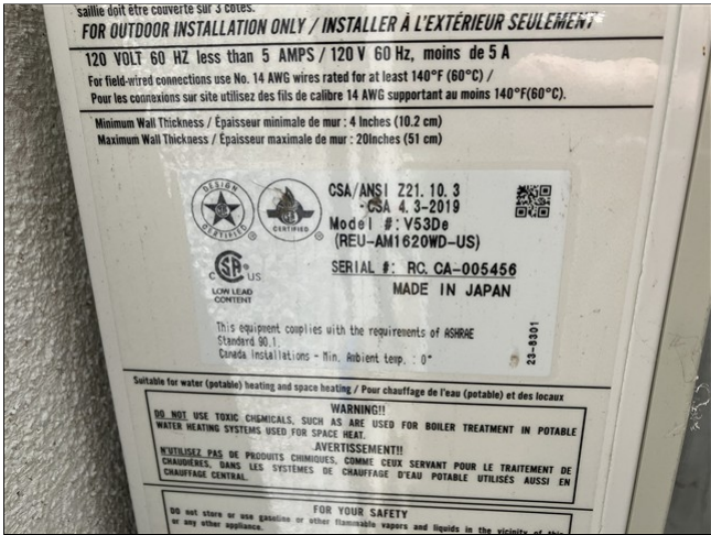
6.2 Item 3(Picture) 1817 tankless water heater
