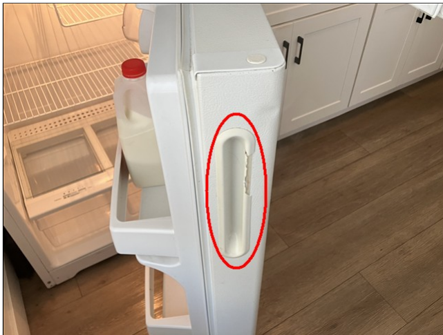
10.7 Item 1(Picture) 1819: fridge handle damage visible
