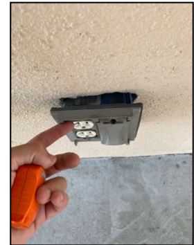
Loose fixture(s) - needs to be serviced
