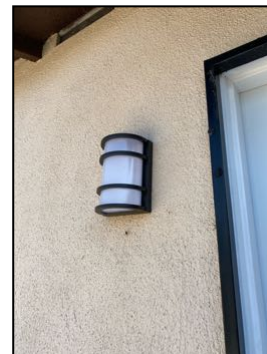
Loose fixture(s) - needs to be serviced
