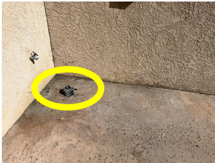
A clean-out is located at the rear.
