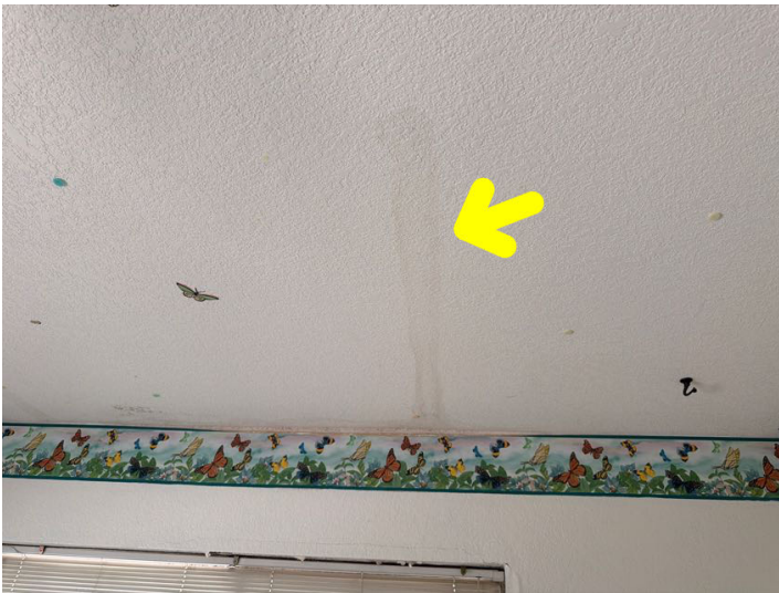
There is a moisture stain on the wall or ceiling that should be explained or explored further.
