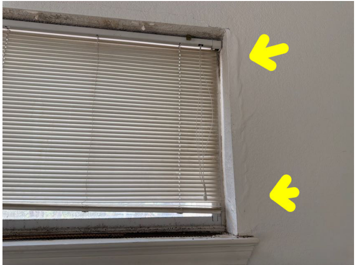
There is a moisture stain on the wall or ceiling that should be explained or explored further.
