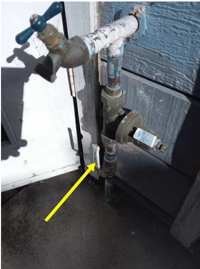
The main water shut-off valve is located at the left side of the house.
