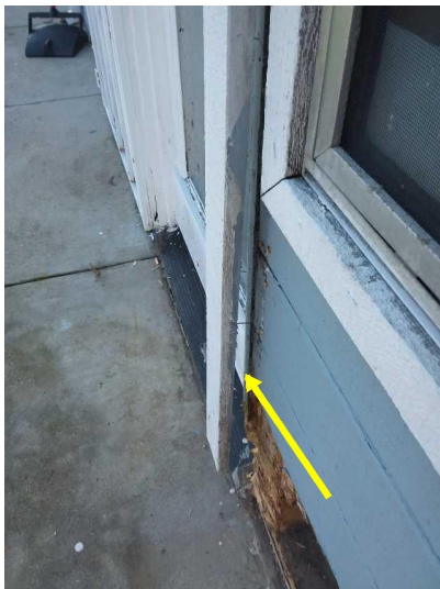
Sections of the fascia board or wood trim are weathered and have separated slightly, and should be serviced to prevent further deterioration.
