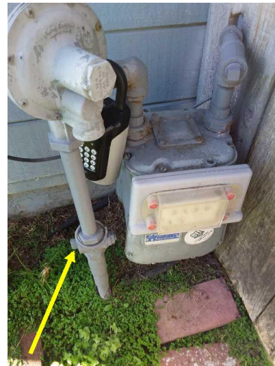
The gas main shut-off is located on right side of the home, unit or building.
