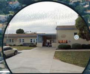
ROSEBANK ELEMENTARY SCHOOL
