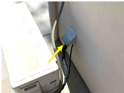
Opening sealed for critter protection
