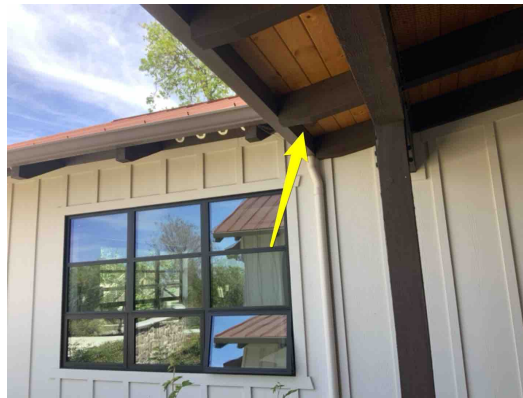
Example - at the front porch cover
