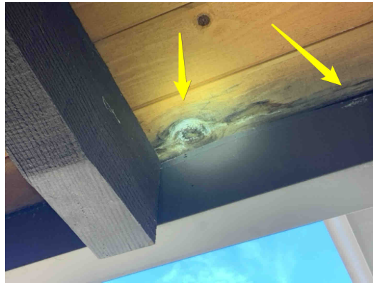
Example - at the front porch cover
