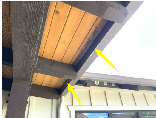
Example - at the front porch cover
