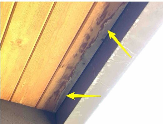
Example - at the front porch cover
