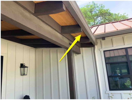
Example - at the front porch cover
