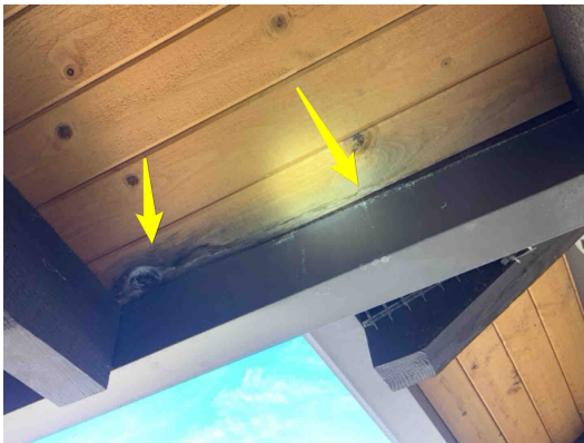
Example - at the front porch cover
