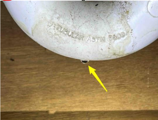
E&C 138: Active leaking from the bathroom sink plumbing: HALLWAY BATHROOM
