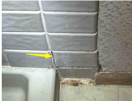
Damaged grout
