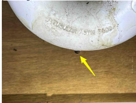
E&C 138: Active leaking from the bathroom sink plumbing: HALLWAY BATHROOM
