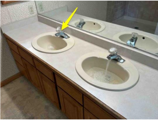
E&C 138: Active leaking from the bathroom sink plumbing: HALLWAY BATHROOM
