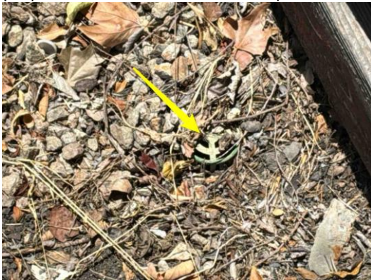
Surface drain warrants attention to Repair And maybe too small
