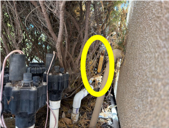
The main water shut-off valve is located at the right side of the home, unit, or building.
