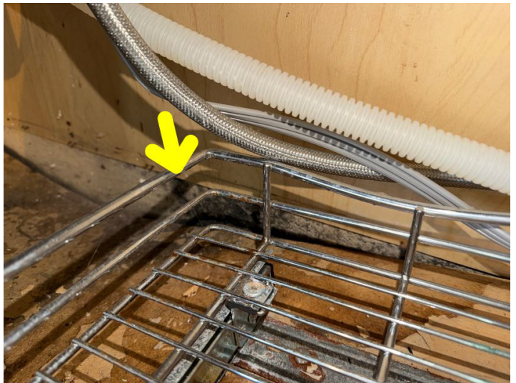
There is a mold-like substance present in the sink cabinet, which should be evaluated by a specialist and serviced as necessary. All molds flourish in a damp environment and many are commonplace, but some are toxic and may represent a health threat.
