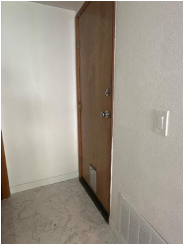
Entrance from garage#1-1.jpg
