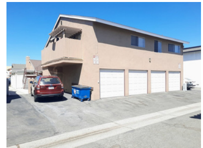
Rear view of garages & Unit D above
