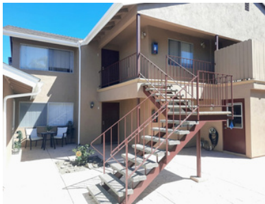
Units B, C, D , laundry room & common area
