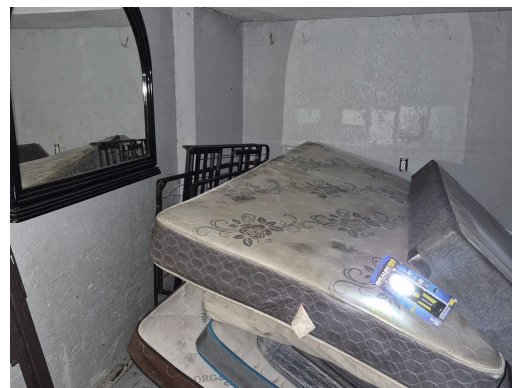
Interior — sound, dry structure; currently used for storage.
