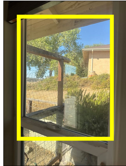
Staining and etching of the glass at the window indicated a loss of thermal integrity.
