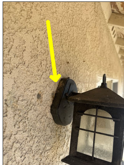
Exterior lighting was loose/not flush to the wall and could expose electrical components to moisture intrusion. rear of the home
