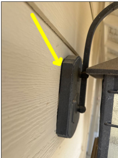
Exterior lighting was loose/not flush to the wall and could expose electrical components to moisture intrusion. front of garage
