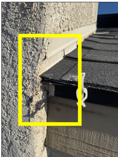
The home had no kick-out flashing installed where walls extended past roof edges.
