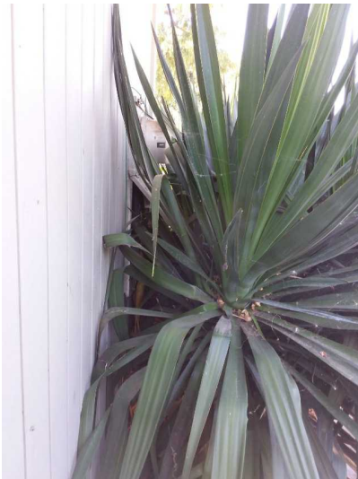
The main panel does not have thirty-six inches of clear space in front of it to facilitate an emergency disconnect, a condition which should be corrected.
