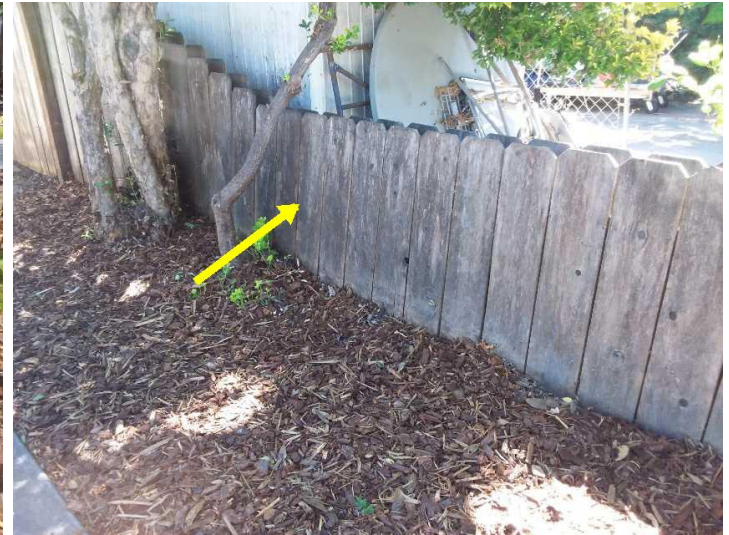
Sections of the fence are leaning or missing which you may wish to have repaired or replaced.
