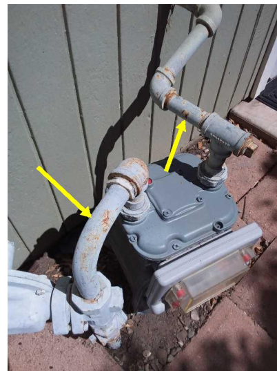
Some of the gas lines at the meter are rusted and should be painted to prevent further corrosion.
