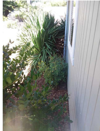
Vines, shrubs or bushes are growing on the house walls and although they are attractive they can introduce pests and rodents and accelerate deterioration. Therefore, you may wish to consider having them removed or cut back to 12 inches away from the home.
