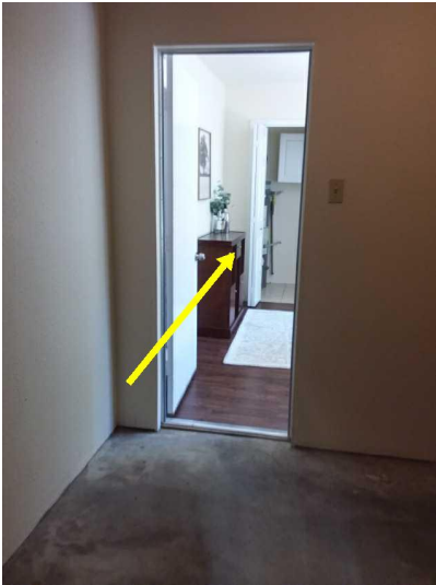
The house entry door is not a fire rated, self-closing and latching door, which should be serviced.
