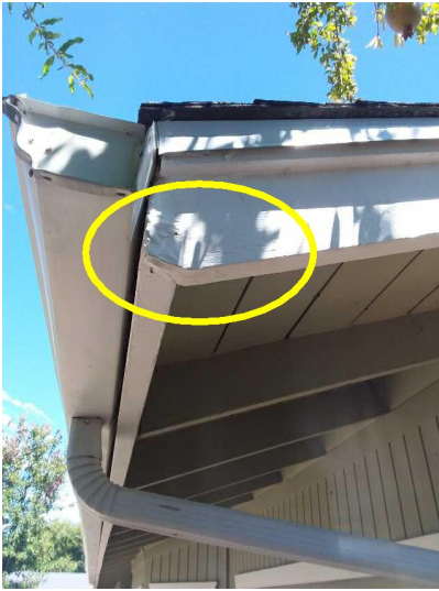
There is damage to the wood trim that should be evaluated by a termite inspector.
