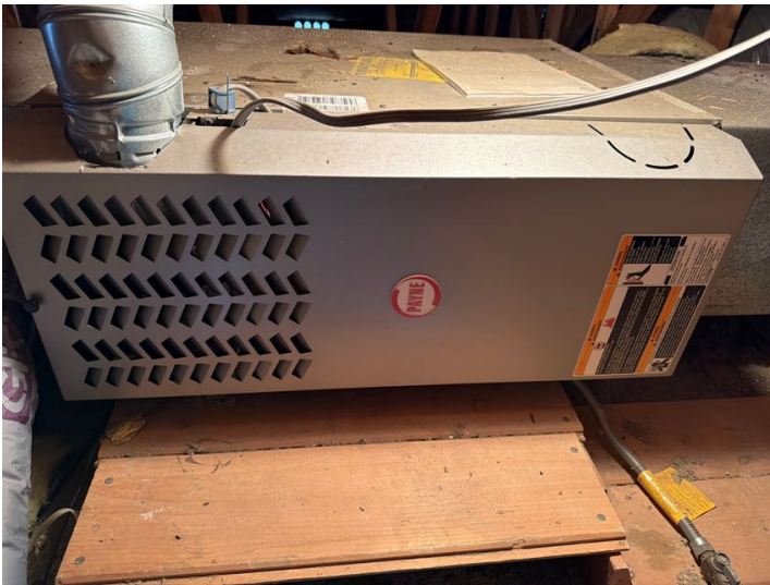
Central heat is provided by a forced-air furnace that is located in the attic.
