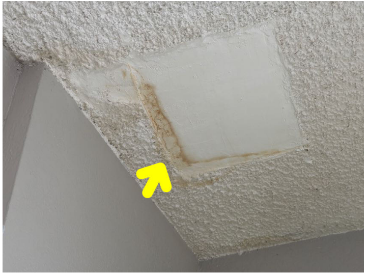
There is a moisture stain on the ceiling that should be explained or explored further.
