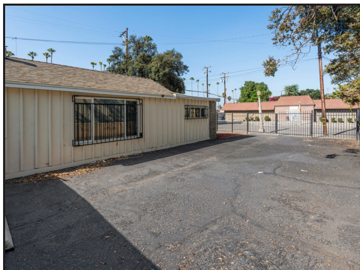
GATED REAR ENTRY AND DRIVE
