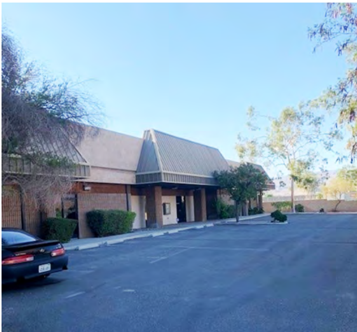
Building Rear Parking
