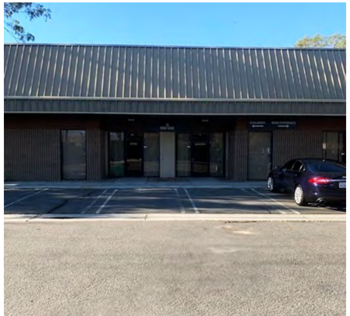
Building Rear Parking
