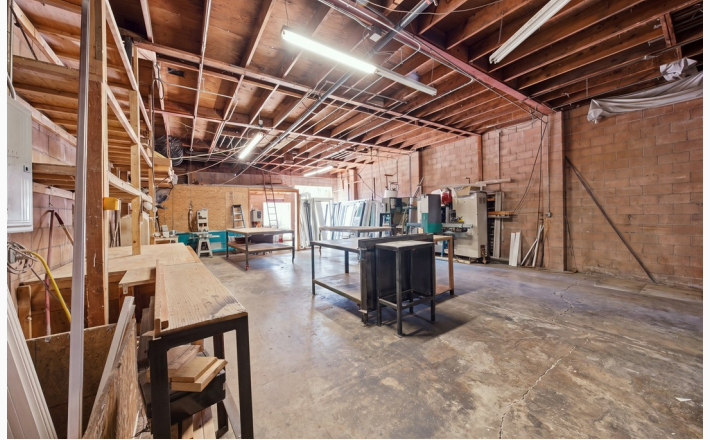
Open work area and clear span under wood truss
