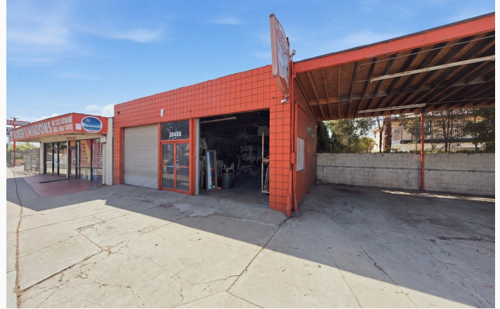
Building and covered parking from Alondra Blvd
