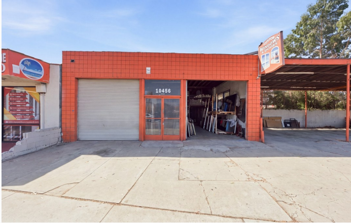
Front elevation and roll-up door on Alondra Blvd
