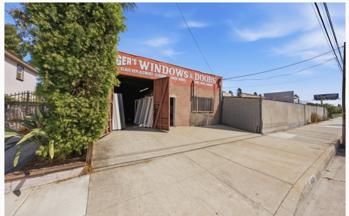
Rear access, gated yard and building signage
