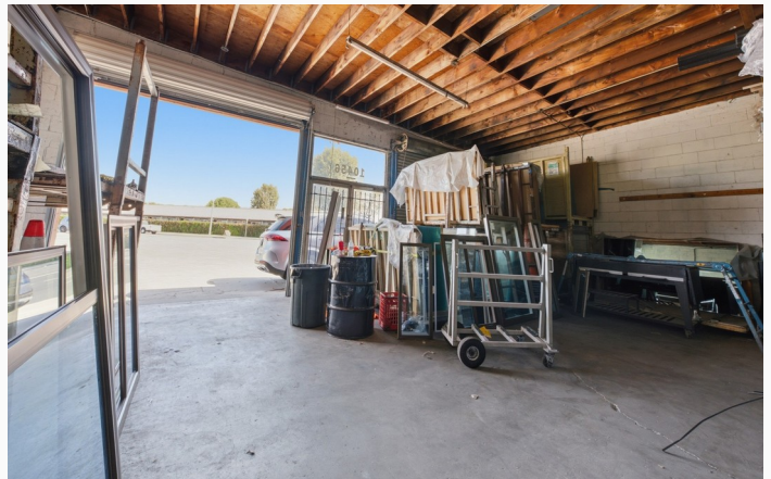
Interior looking out through the roll-up door
