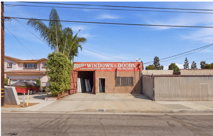
Rear elevation and secured yard from Trabuco St
