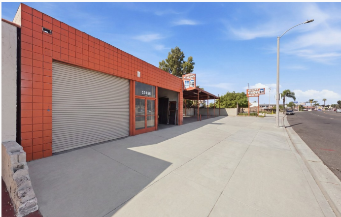
Frontage and drive approach along Alondra Blvd
