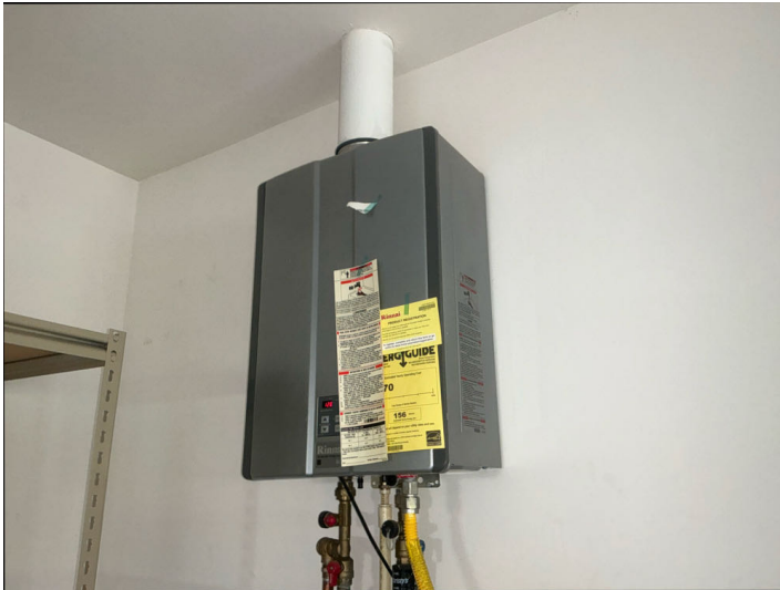
The residence is served by a tankless water heater located in the garage.
