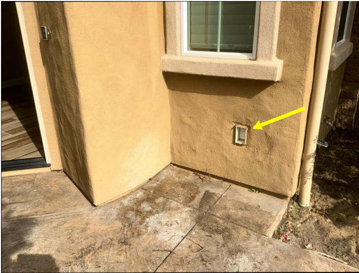
Some of the exterior electrical outlets do not have a weather rated cover or the cover is damaged and should be serviced.
