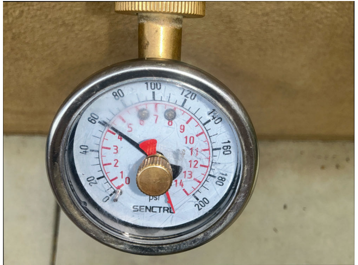
A functional pressure regulator is in place on the plumbing system.
