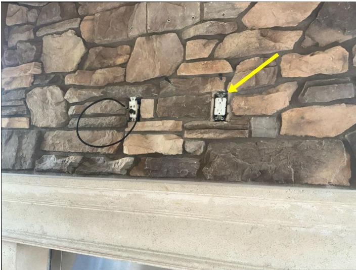
Some of the exterior electrical outlets do not have a weather rated cover or the cover is damaged and should be serviced.
