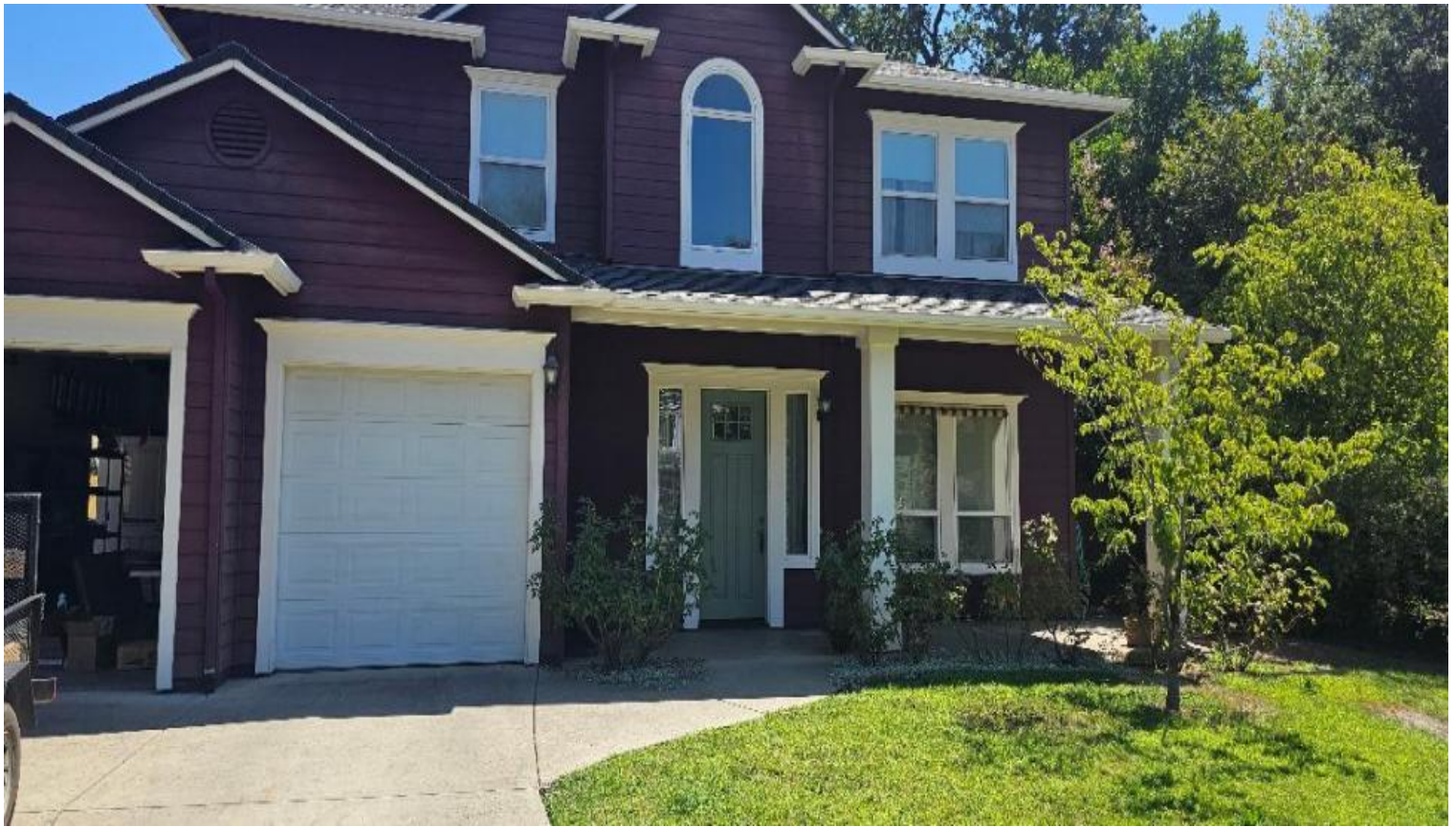
Front of the structure.
