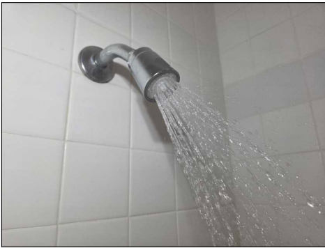
Shower fixture(s) tested and operated
