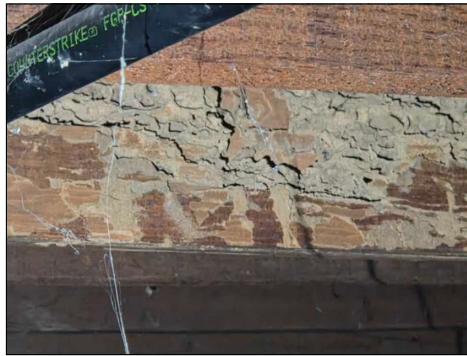
Heavily deteriorated joist in areas - needs to be serviced/further evaluated by a specialist
