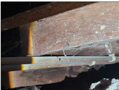
Heavily deteriorated joist in areas - needs to be serviced/further evaluated by a specialist
