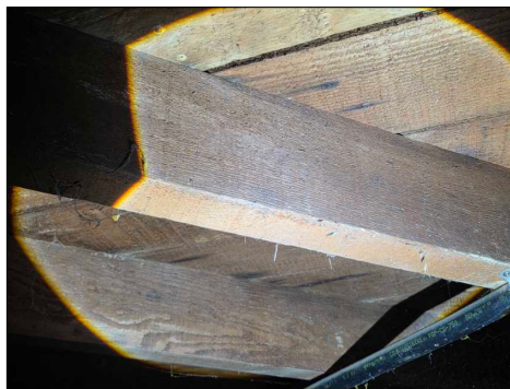
Heavily deteriorated joist in areas - needs to be serviced/further evaluated by a specialist
