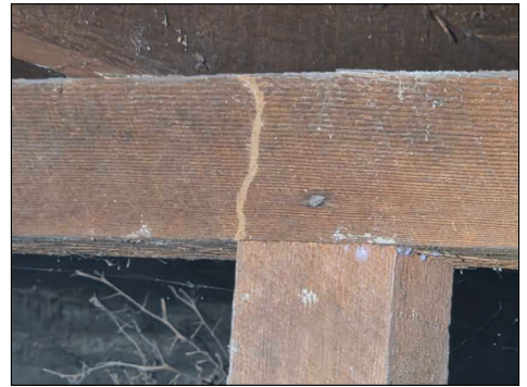
Missing brackets at attachment points - recommend upgrade
