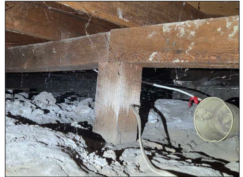
Missing brackets at attachment points - recommend upgrade
