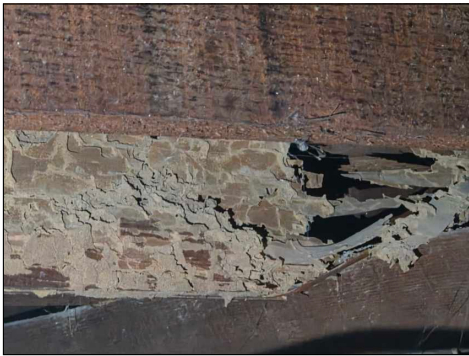
Heavily deteriorated joist in areas - needs to be serviced/further evaluated by a specialist
