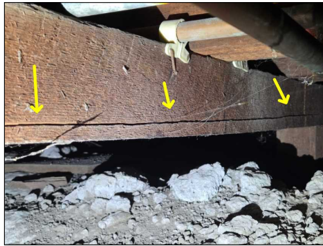
Cracked/sagging girder - needs to be serviced
