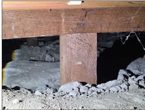
Cracked/sagging girder - needs to be serviced
