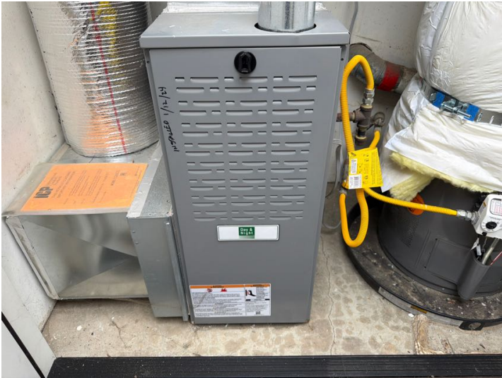
Central heat is provided by a forced-air furnace that is located in an exterior closet.
