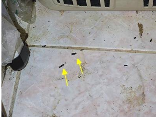
Photo 1-2 Closet below the stairs
