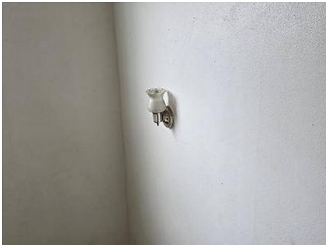
Photo 48-3 At the stairs
