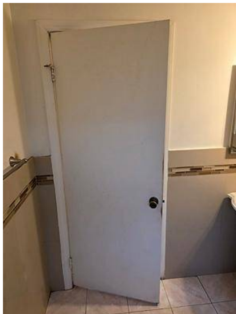
Photo 97-1 Bathroom, 1st floor
