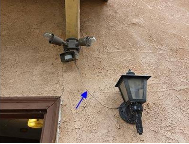
Photo 35-1 Front of unit
