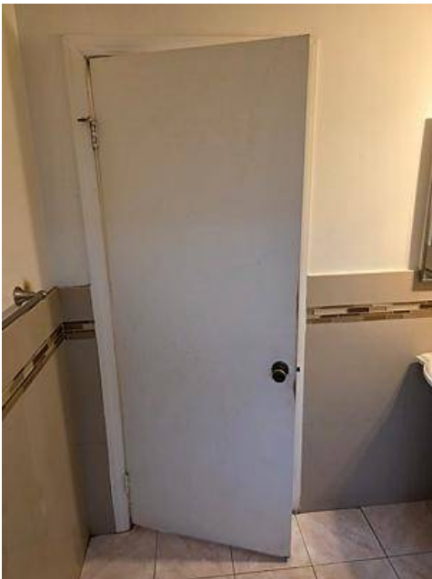
Photo 97-1 Bathroom, 1st floor
