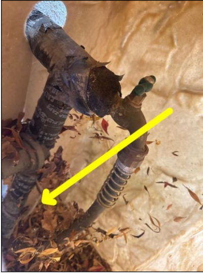
Main water shut off to the home where the main line enters the home.
