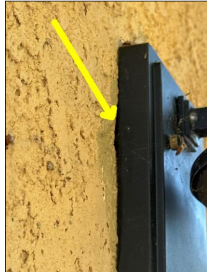
Exterior lighting was loose/not flush to the wall and could expose electrical components to moisture intrusion. front of garage
