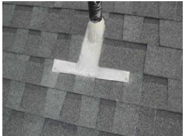
Seal the nails at the base of the flashings.
