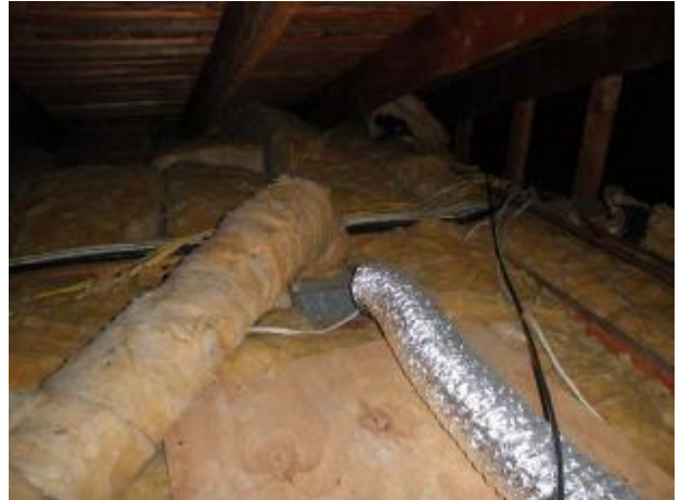
Bathroom exhaust fans vent directly into the attic.
