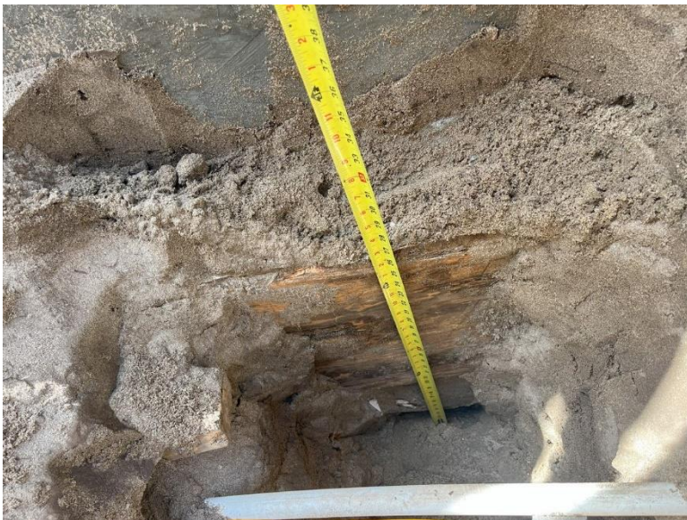
Photo 4: New Footing (Embedment Measurement – ~3'-0")
