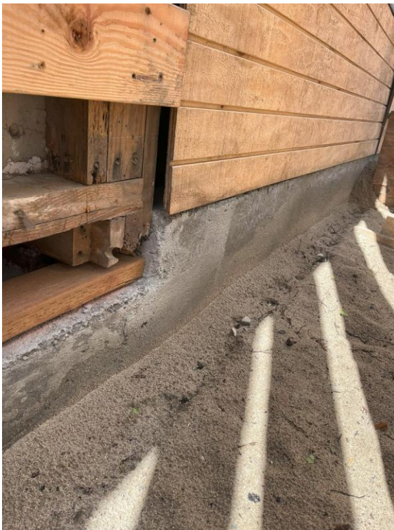
Photo 2: New Footing at Side of House
