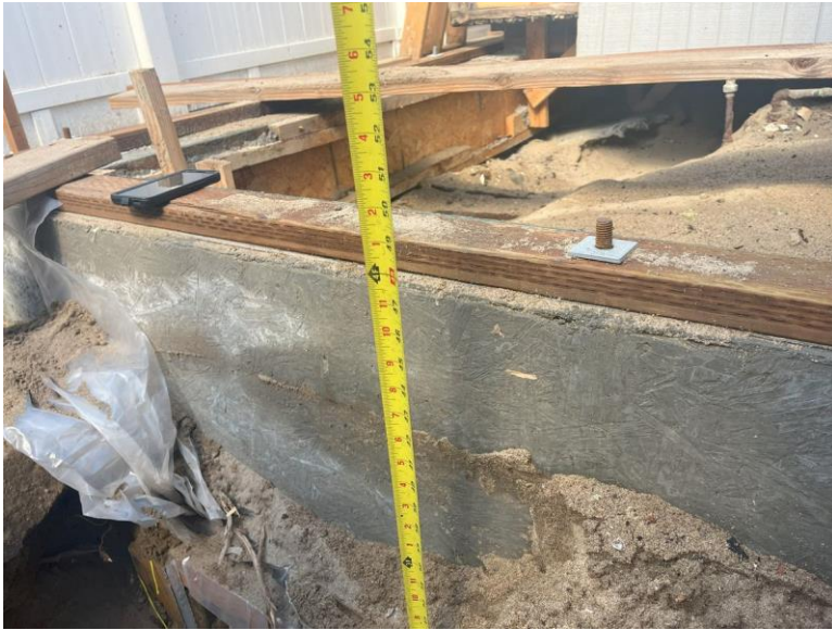
Photo 3: New Footing (Total Depth Measurement – ~4'-0")
