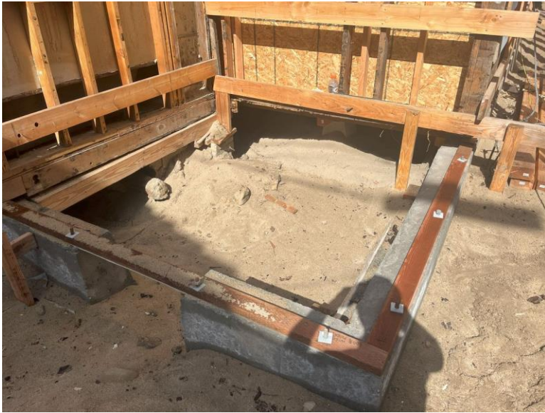
Photo 1: New Footing at Rear of House (Overview)
