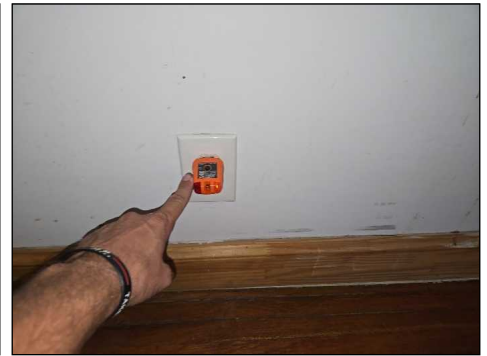
Non-energized (dead) outlet(s) - needs to be serviced
