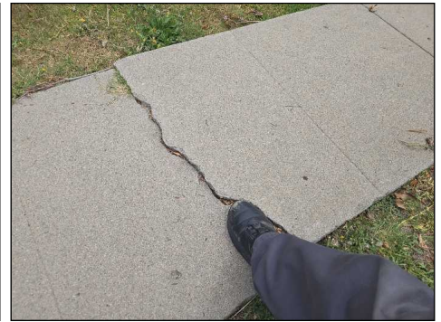
Moderate cracking in areas - recommend maintenance and patching as needed
