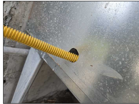
Flexible connector through sheet metal cabinet - needs to be serviced
