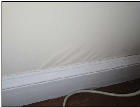
Peeling/blistered/cracking paint in areas
