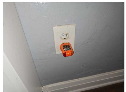
Non-energized (dead) outlet(s) - needs to be serviced
