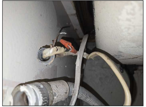
Exposed connections - potential hazard - needs to be serviced
