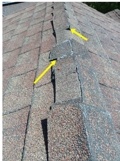
The roof has one or more damaged or missing shingles that should be repaired by a licensed roofing contractor.
