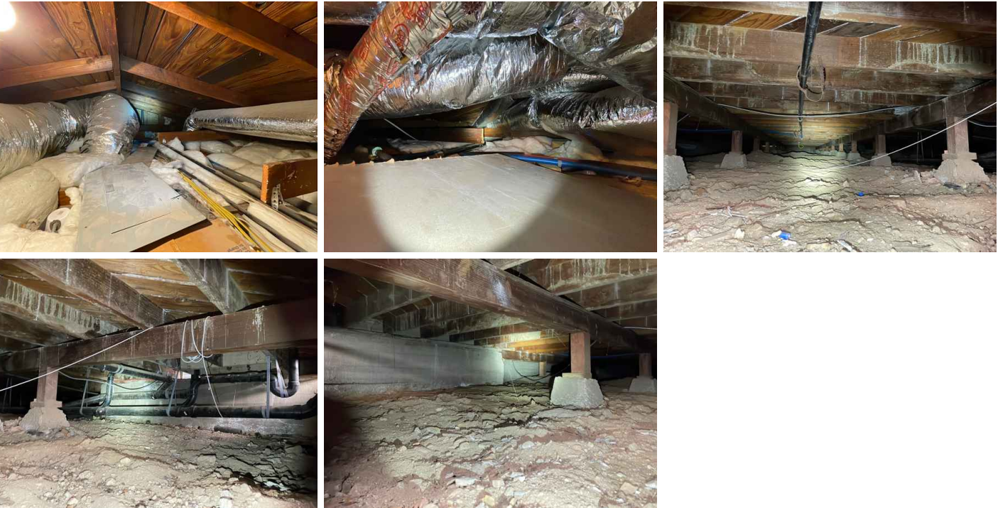
General: Method to observe the attic Inspected from entrance
