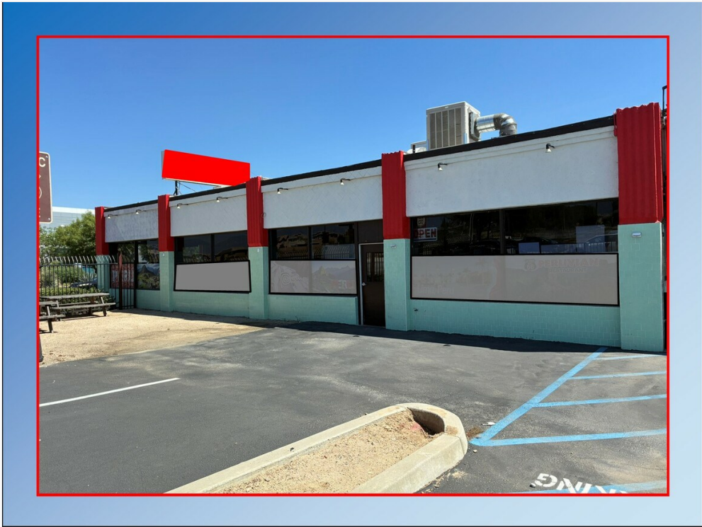
Front Pic of Building 4
