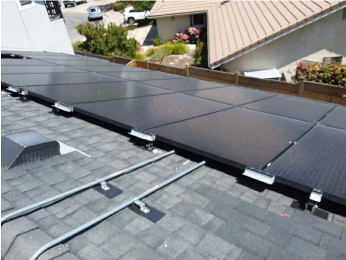
17 panels on lower rear roof
