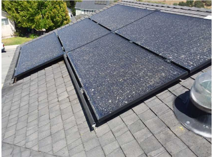
5 panels on upper front roof
