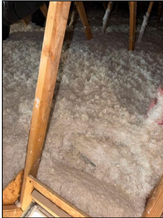
36. Blown-in Fiberglass
