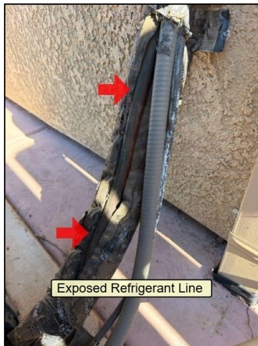
35. Insulation Damaged
