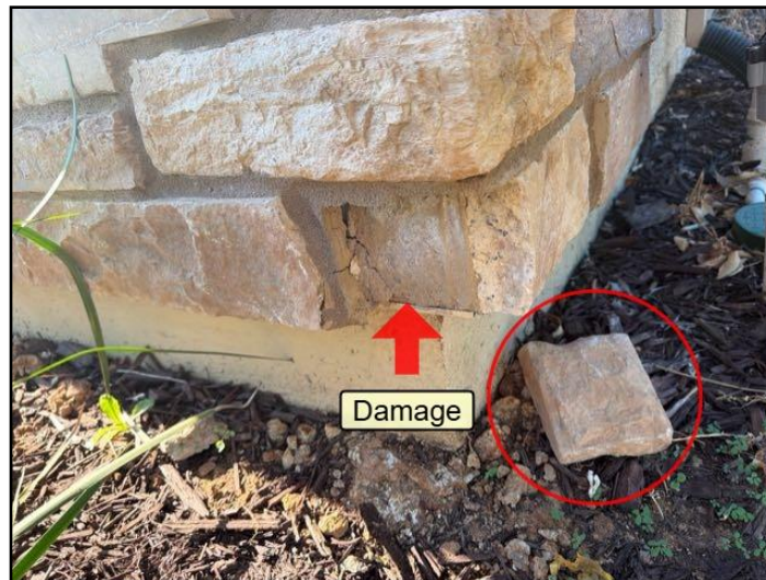
15. Mechanical damage
