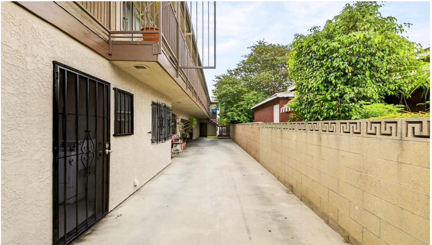
Side walkway to ground-floor units
