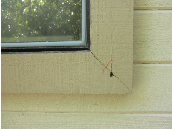
Moisture damage to the wood trim at the window in the laundry closet.
