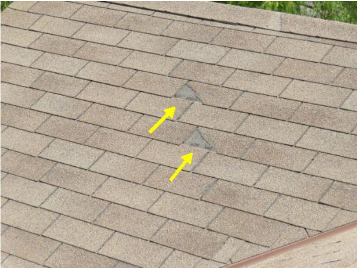
missing shingles
