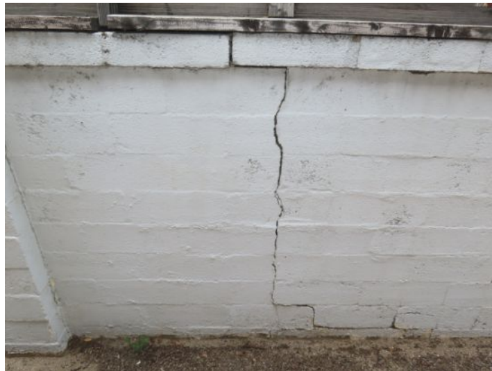
separating cracks
