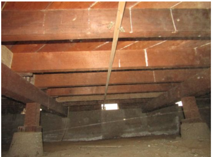
deteriorated wood in areas
