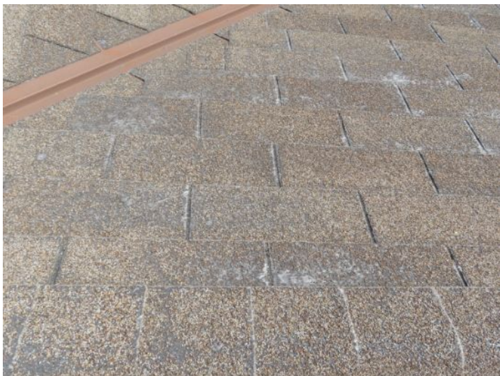
deteriorated roofing material
