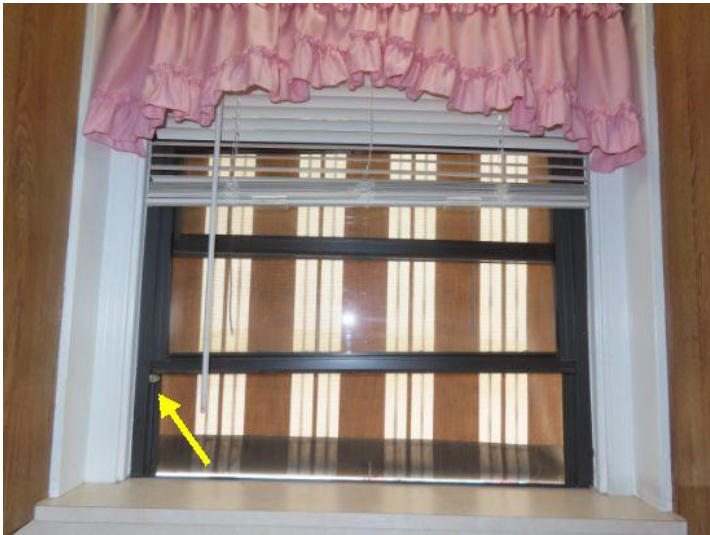
loose balance spring at the window
