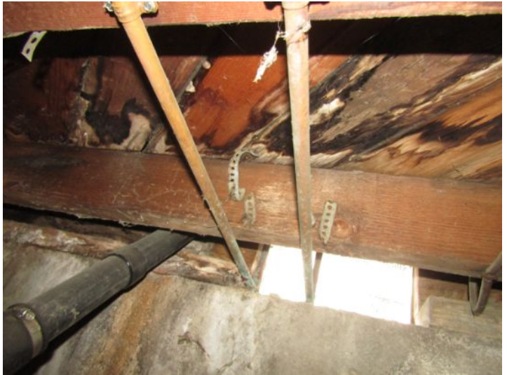
deteriorated wood in areas
