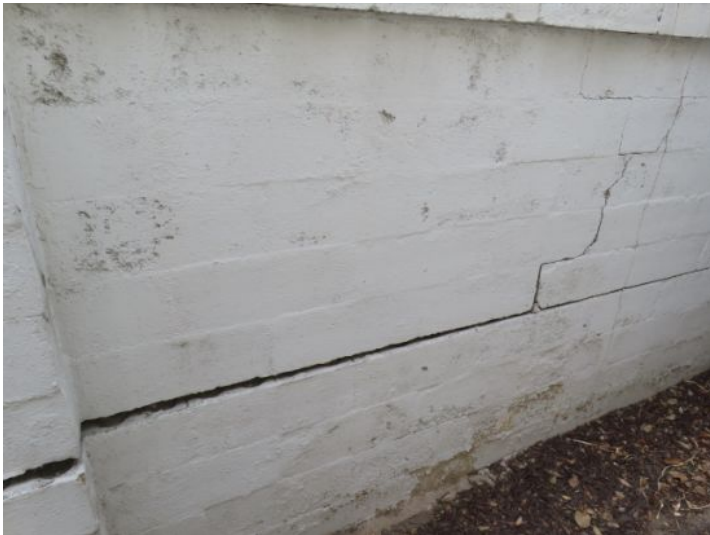
separating cracks
