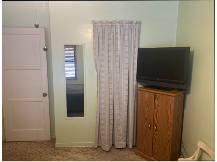
closet door is missing
