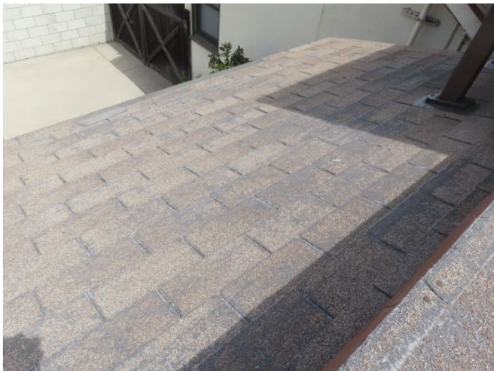
deteriorated roofing material
