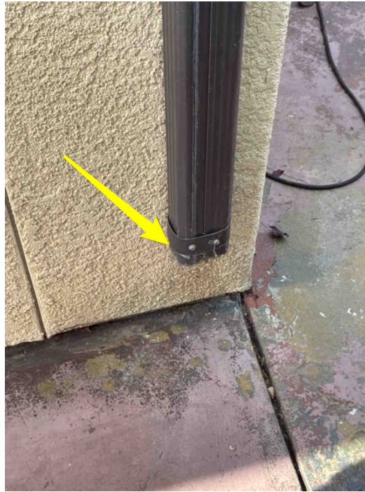
Example. On the southeast corner
