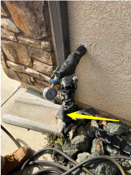
Shut off valve location
