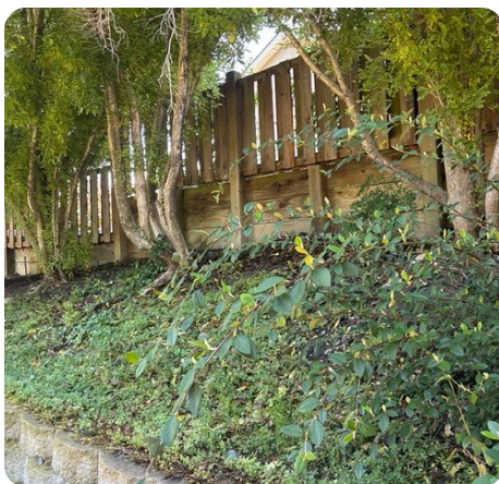
Functional wooden retaining wall at rear property edge.
