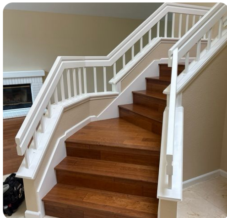
Stairwell railing installed on pony wall.
