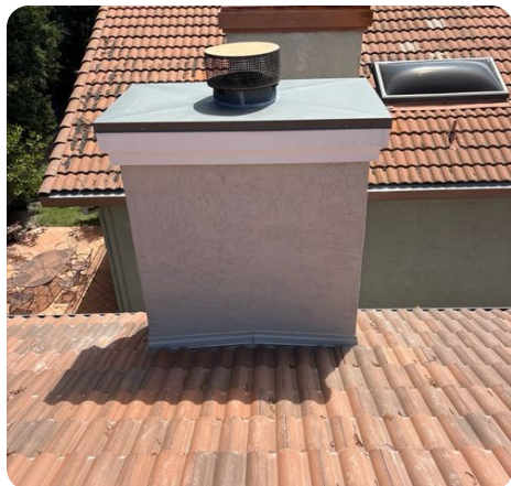
Family room fireplace chase as viewed from upper roof surface.
