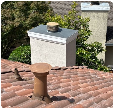
Living room fireplace chase as viewed from upper roof surface.
