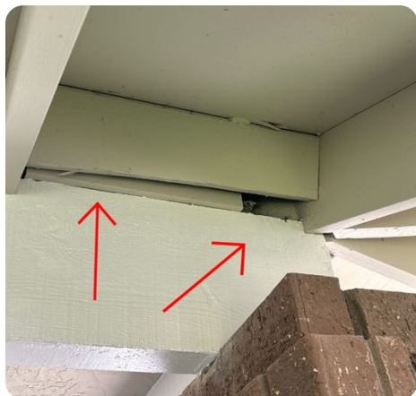
Open soffit blocking at main entry porch cover.
