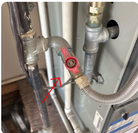
Natural gas control valve serving furnace.
