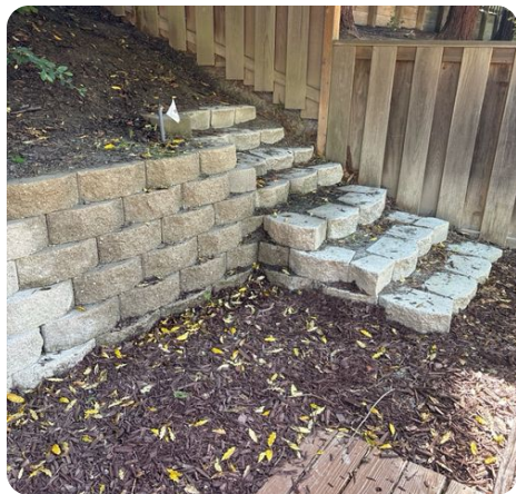
Functional masonry, retaining wall.
