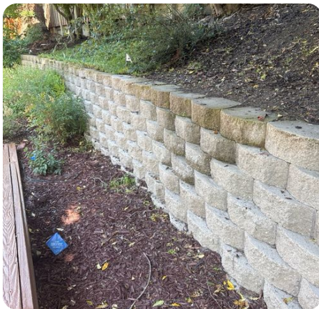
Functional masonry retaining wall. Good morning how are you?
