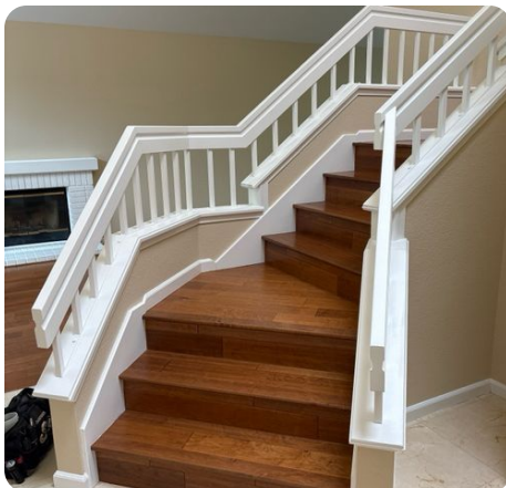
Stairwell railing installed on pony wall.
