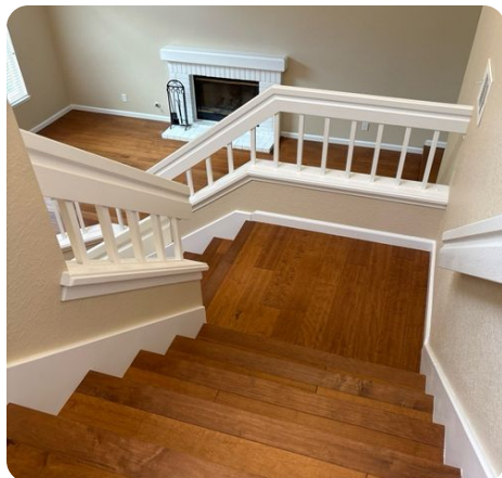
Stairwell railing installed on pony wall.
