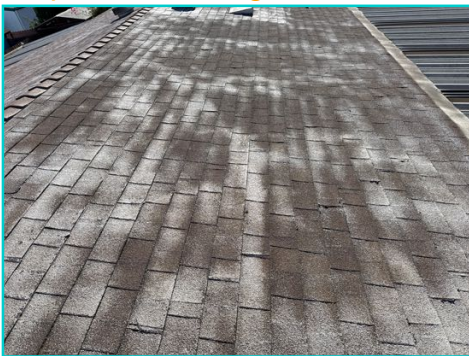
deteriorated shingles
