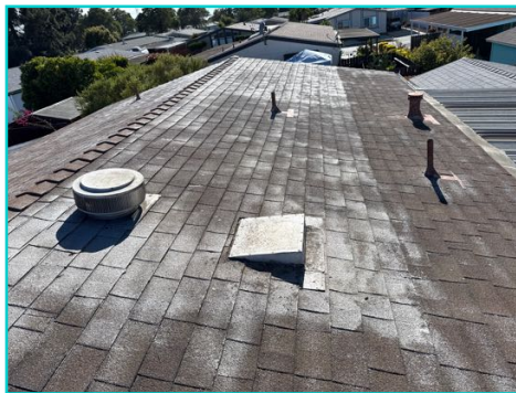
deteriorated shingles
