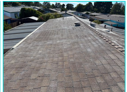
deteriorated shingles
