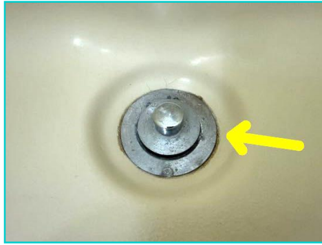
corrosion here
