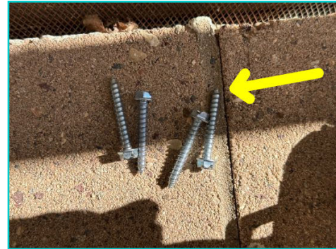
improper pointed screws
