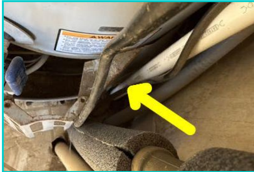
improper termination
