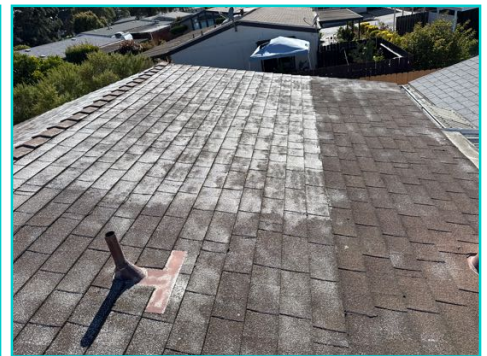
deteriorated shingles
