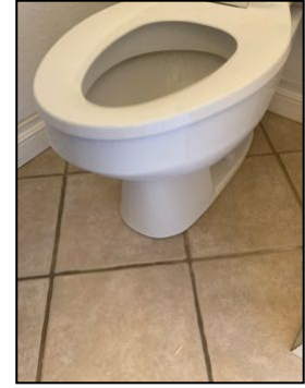
Toilet loose at floor - needs to be serviced at upstairs master, downstairs half bathrooms
