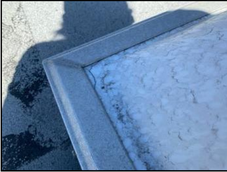
Cracked lens - small - over master bathroom - recommend service/sealing/patching
