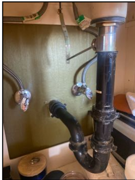
Heavy silicone used under sink at drain/connections - evidence of past leaking - recommend evaluation at upstairs master bathroom
