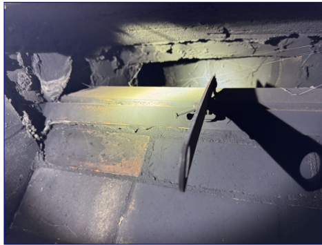
Fireplace Fireplace Lintel, Damper, Firebox
