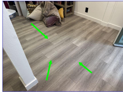
Interior Areas Flooring Condition
