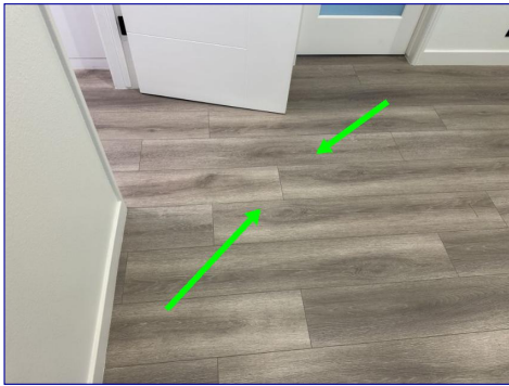
Interior Areas Flooring Condition
