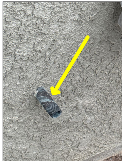
This pipe is the drain for the fire sprinklers when they are tested
