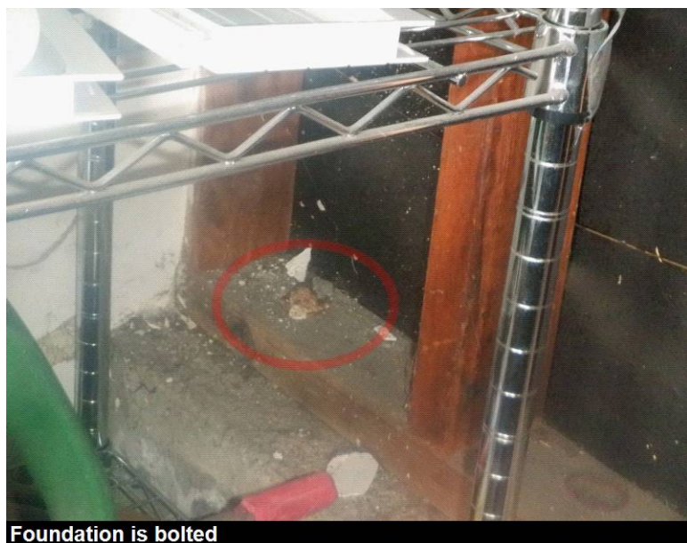
Foundation is bolted
