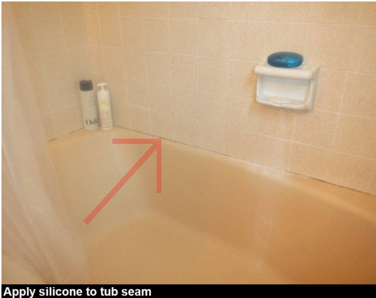
Apply silicone to tub seam
