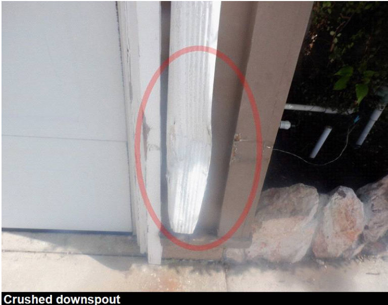
Crushed downspout
