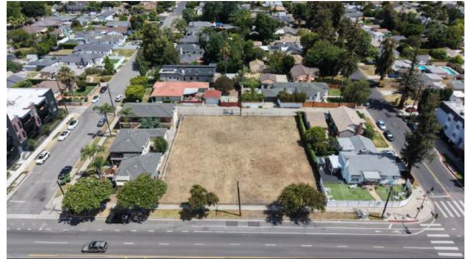
Site Perspective Facing North — Cleared and Ready for Construction
